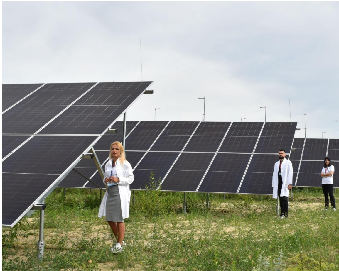
CREATEGREEN – new solar power plant
