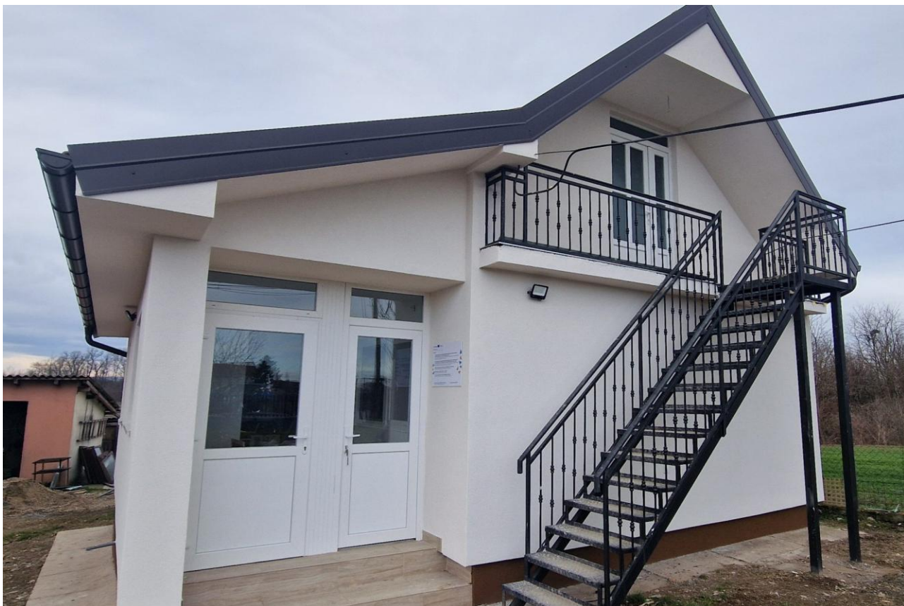
SOCCARE - premises in Jelenča, Vladimirci, and Šabac were adapted and equipped
