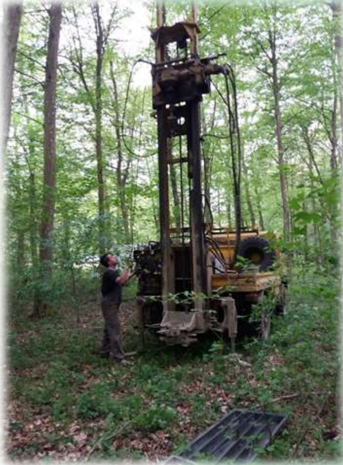
Drilling of a piezometric well
